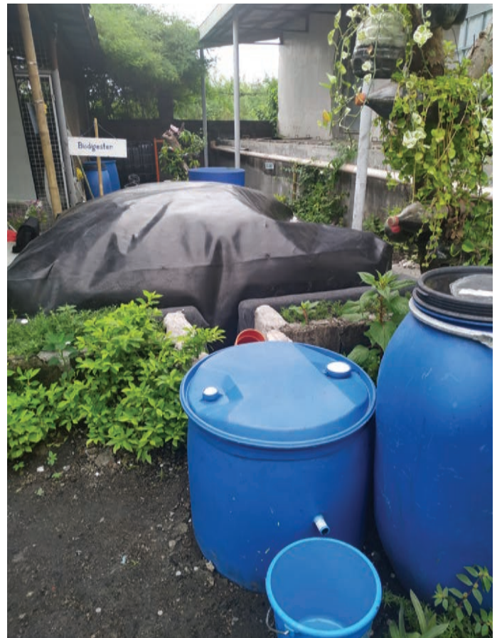
▲ The six-cubic meter biodigester system
